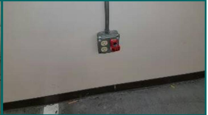
No power to outlet at first floor left side lab
