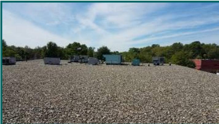
7 rooftop package units, 1 roof top mounted compressor for ductless split and 1 rooftop compressor for split system
